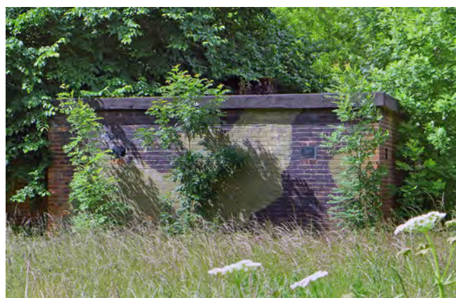
Many of the buildings still have their camouflage visible (or not visible!)
